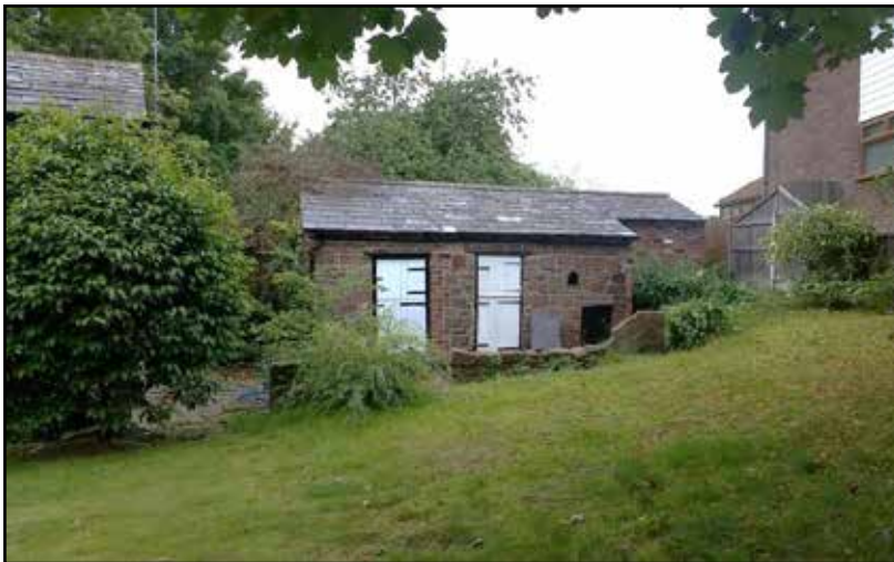
Figure 14 – Outbuildings at Sunnyside Farm, built using sandstone, likely to be from the former quarry on Pex Hill.
