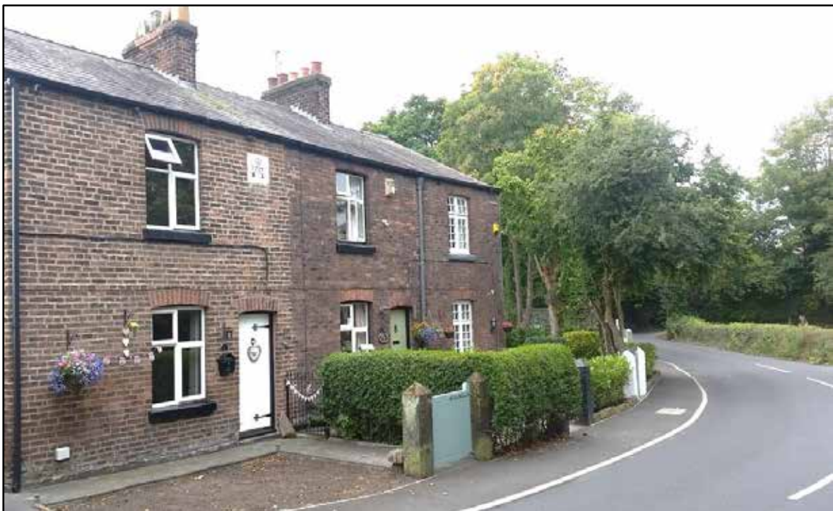
Figure 16 –Town End Cottages, date from the 19 th century of brick laid in common bond.
