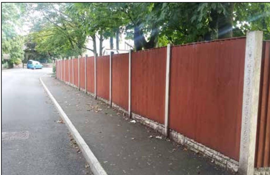
Figure 7 – Tall wooden fencing creates an imposing inactive frontage that detracts from the wider natural setting of the conservation area at Hall Lane.
