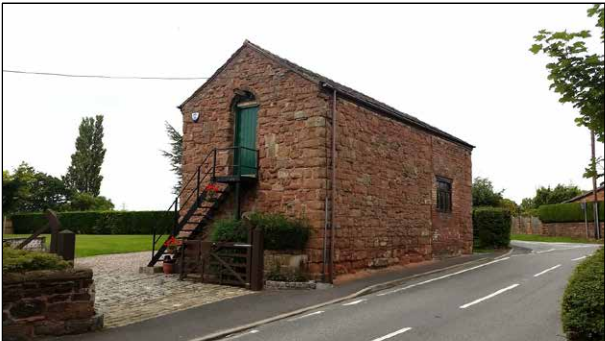
Figure 11 – Example of former agricultural building typical of the conservation area, in the local vernacular style using local stone.
