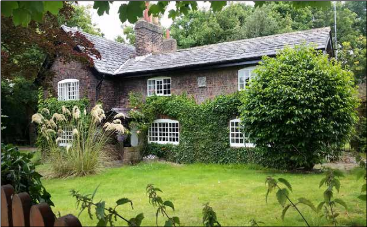
Figure 12 – Typical early horizontal sliding sash windows with small panes, few original windows remain within the conservation area with many significantly altered.
