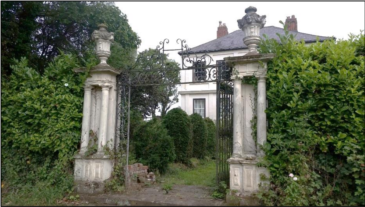
Figure 4 – Cronton Hall’s Grade II listed wrought iron gates, dating back to early 18 th century with Cronton Hall partially visible in the background.
